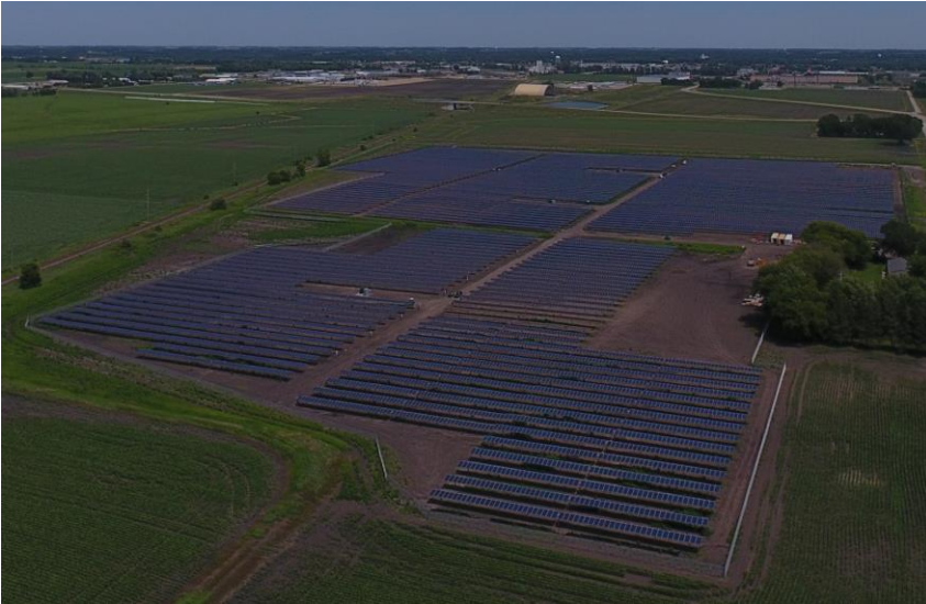
Southern Minnesota Municipal Power Agency's 5 MW Lemond Solar Station Owatonna, MN
