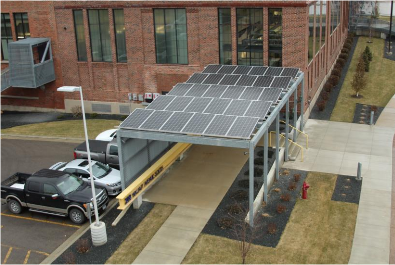
Owatonna Public Utility's 10 kW Demonstration Solar Owatonna, MN
