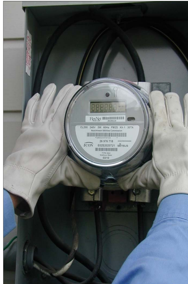
An AMI meter that was just installed.
