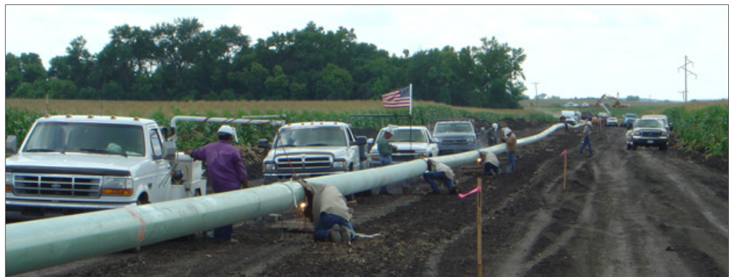
Men at work on the pipeline.
