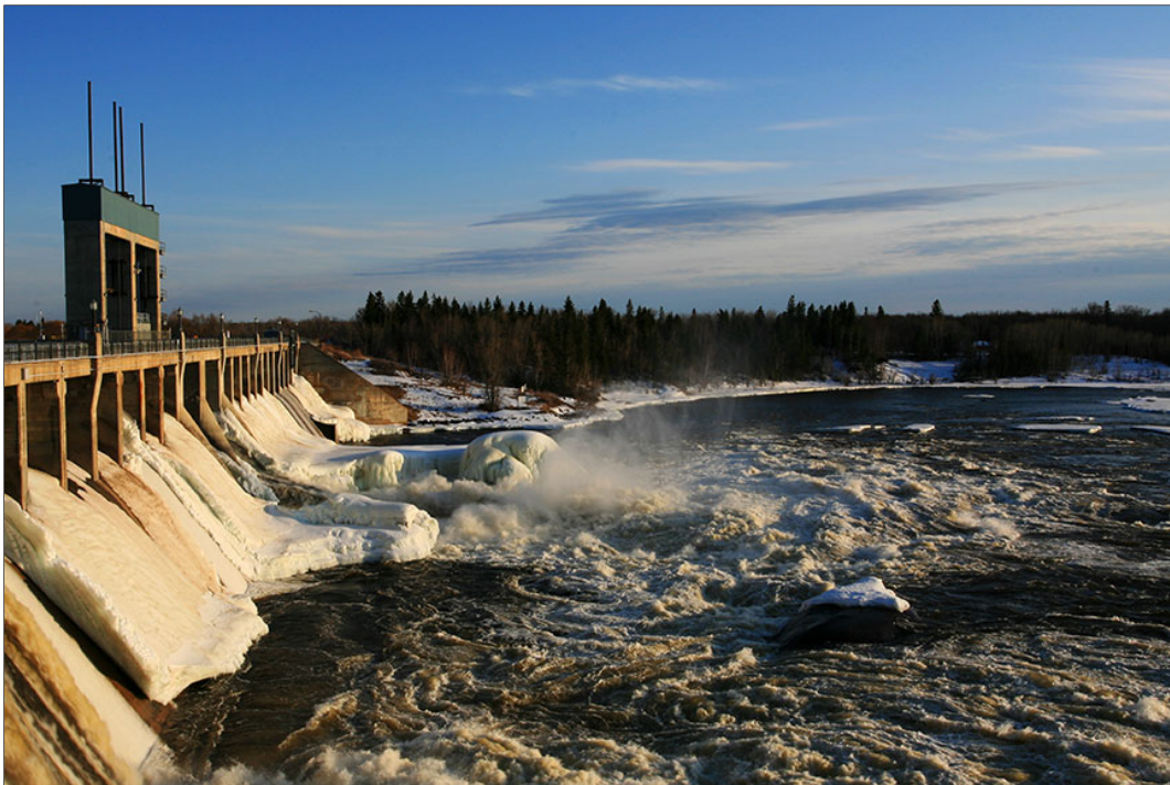
A modern-day picture of the Manitoba Hydroelectric dam. This photo is courtesy of flickr.com.
