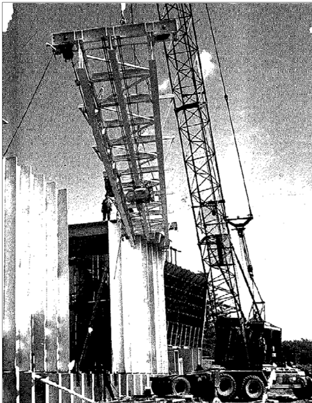
Expansion construction at the downtown plant.
