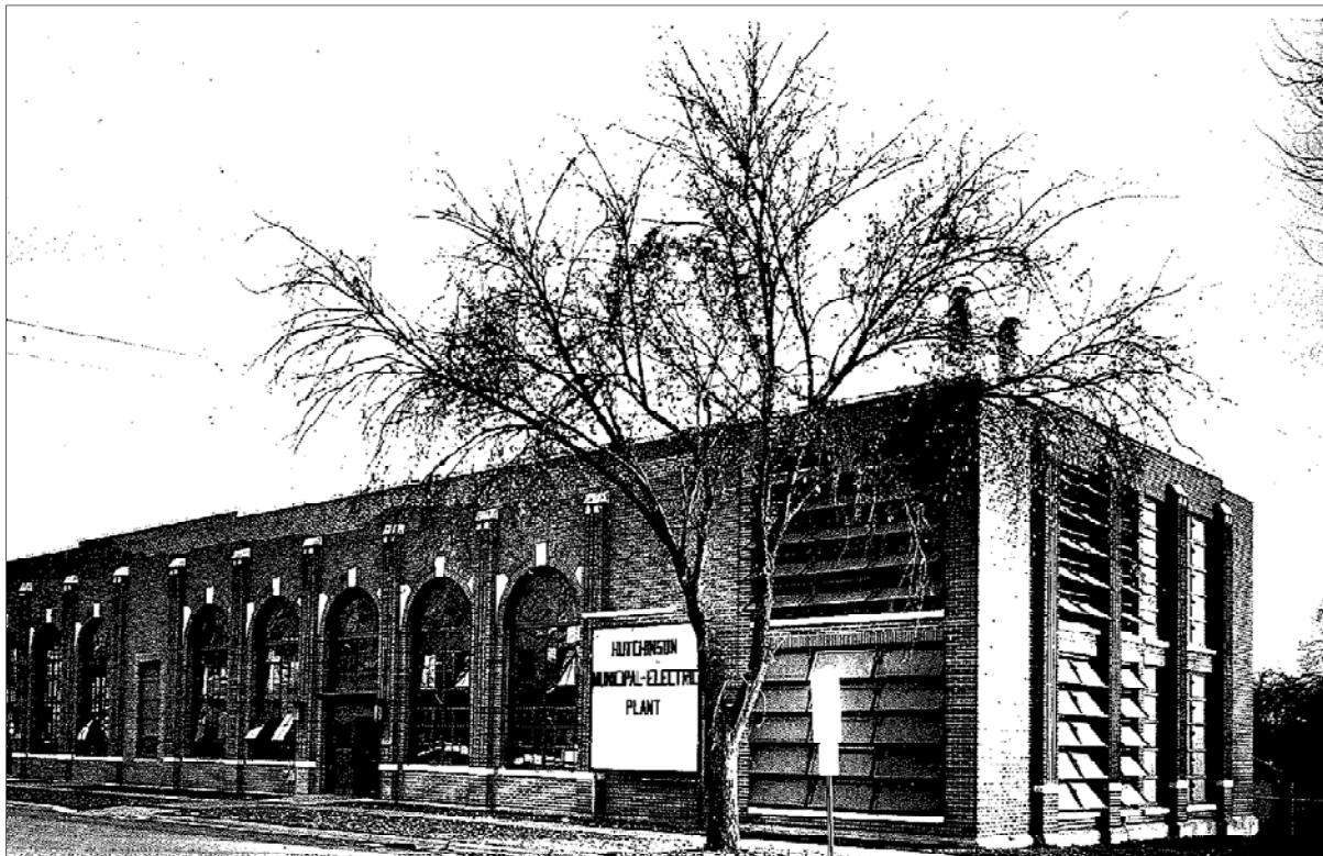
The Electric Plant at the end of the 1950s.
